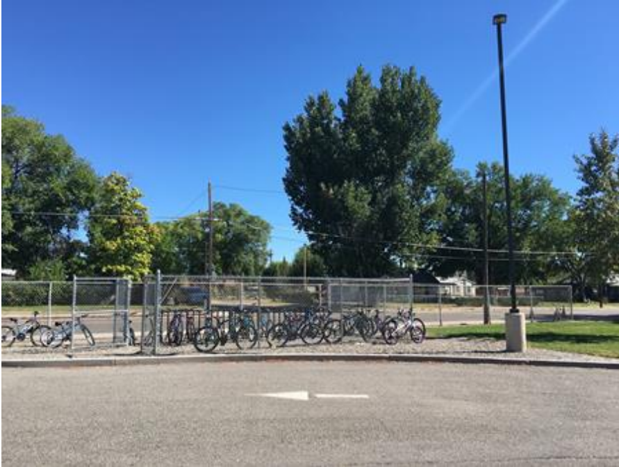
Figure 2: - Lighting does not illuminate bike cage on east side of school.
